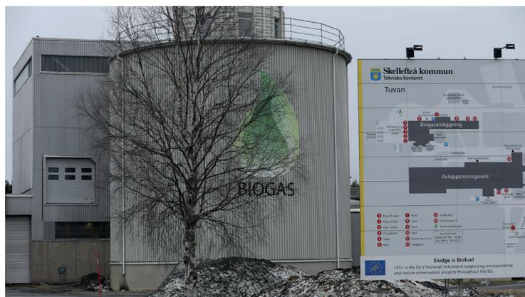
Contrary to the Swedish "co-digestion" terminology used, Tuvan's food waste biogas plant is a co-located facility and separate from the WWTP. Shared facilities, biogas storage, upgrading, compression and flare are all post-digestion.
