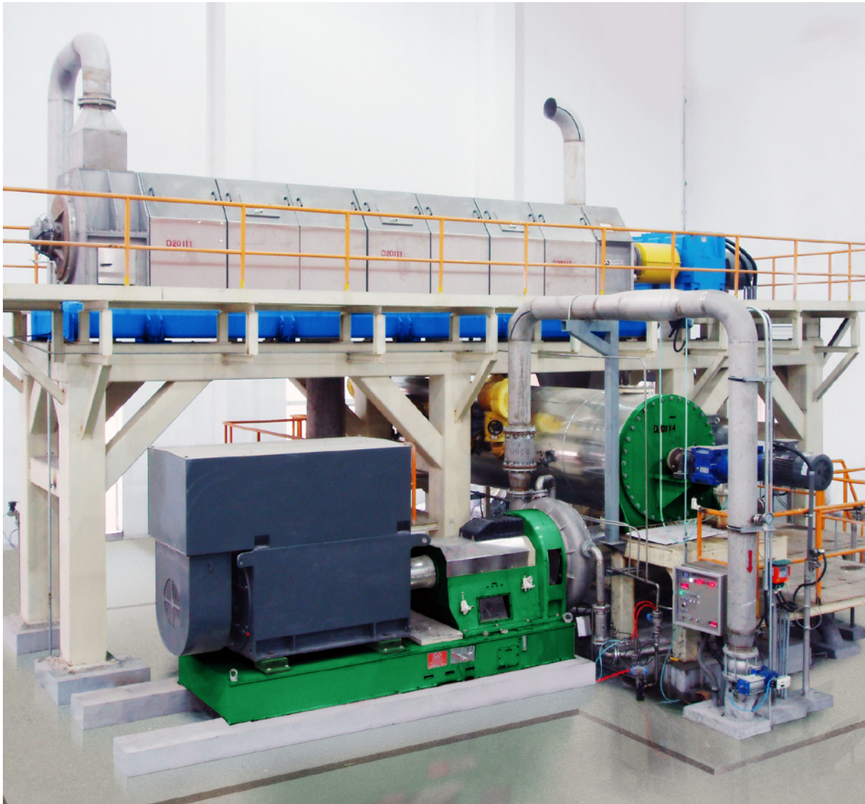
Krima HDS installation.
